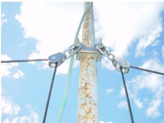
This is a view of the modified truss system using pulleys mounted on the mast. This is done to put the turnbuckles down lower within reach for adjustment. Phillystrand is used for the truss cables. The pulleys and associated hardware are all stainless steel. (The system was originally designed by Robert Polinski, KD5YVQ.)
