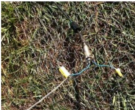
Step 3. Get some local chicken wire (any hardware store in US and in most 3<sup>rd</sup> world countries.) lay it out in a cross fashion (2 ft X 25 foot times two) At the intersection wire tie the two pieces together and make a short piece of the wire to stand up so you can use it to connect to the ground side of the antenna (your chicken wire used as radials)
