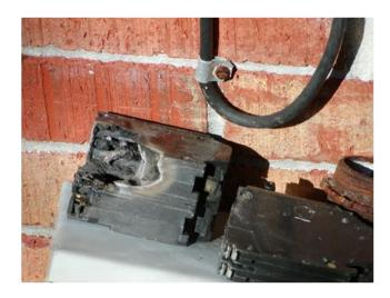
This is the circuit breaker that failed and burned up my feed panel. The coax is my computer modem feed which just happens to be in the picture.
