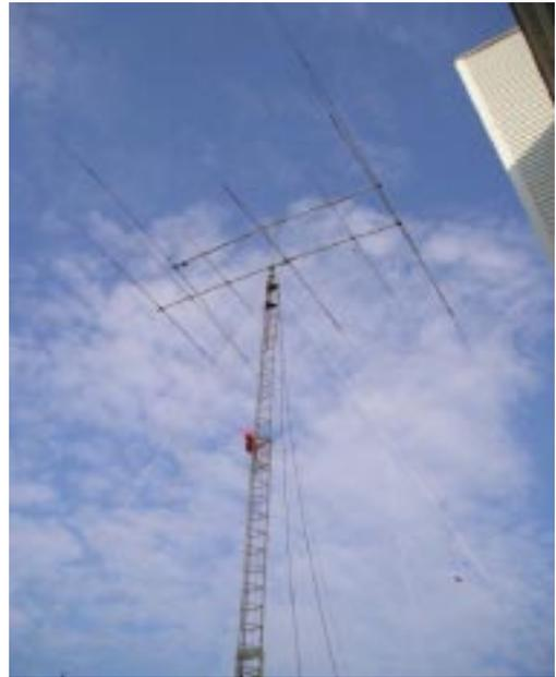
The SSB station tower with TH-6-DX and 2 el 40 at about 50 ft.
